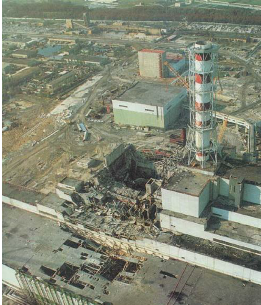
Chernobyl reactor number four after the disaster, showing the extensive damage to the main reactor hall (image center) and turbine building (image lower left)
